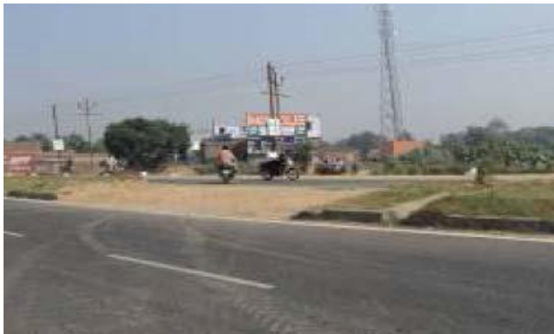
Figure : Unauthorized Median Opening at Km 232.050
