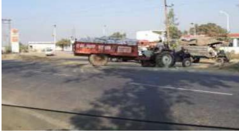
Figure . Unauthorized Median Cut at Km 226.300:
