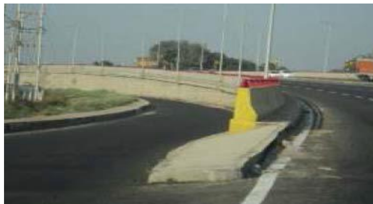
Figure .Service Road & Start of Underpass
